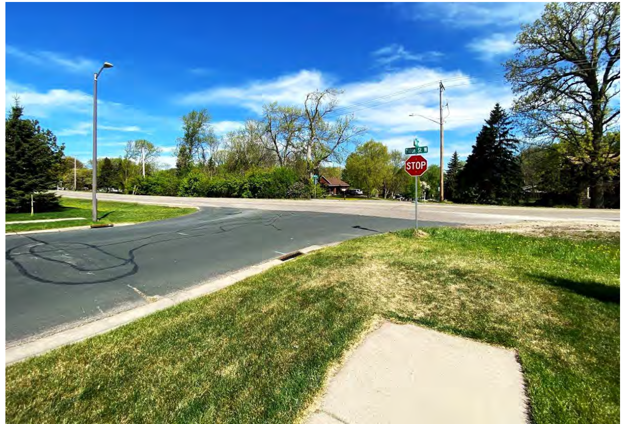
Italy Avenue looking north at 210 th Street with the existing sidewalk shown. Source: SRF Consulting Group, 2020
