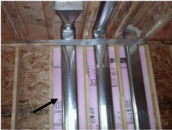
7. 1 ½ rigid foam insulation used behind heat runs in exterior walls.
