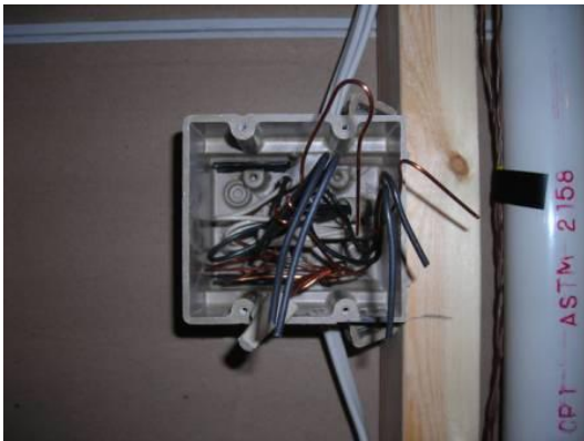
1. Electrical rough-in have all boxes made up and ready with minimum 6-inch tails.
