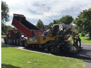
Installation of new asphalt surface
