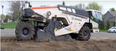
Reclamation of existing asphalt
