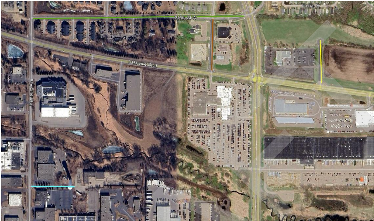
Figure 1-3. Existing roadway layout showing 214th Street West (light blue), 210th Street West (green), Glade Avenue (brown), and Gateway Drive (yellow).
