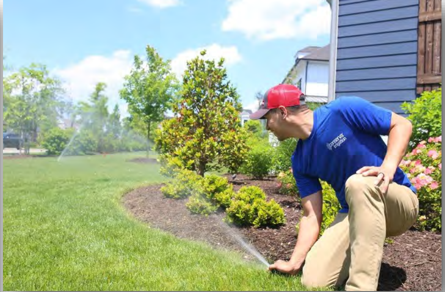
(Right) All audits found that the most profound water savings can be achieved by scheduling monthly system walk-throughs to catch breakages that can be missed due to early morning or late night operation times.
