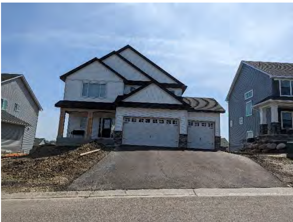
Berres Ridge Single-Family – Under Construction
