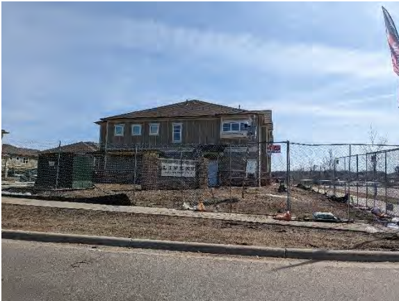
Livery Modern Apts. – Under Construction
